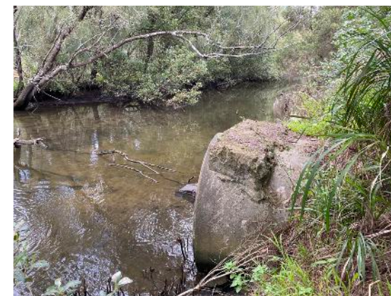
Damaged concrete inlet pipe empties directly into southern Scarborough Pond
