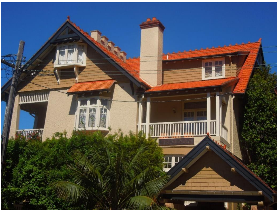
(‘The Hastings’, c.1905, in Neutral Bay survives as one of the best examples of Jackson’s work and an embodiment of the Arts and Crafts aesthetic with its varied palette of materials and its many elements. Photo by the author, 2015)
