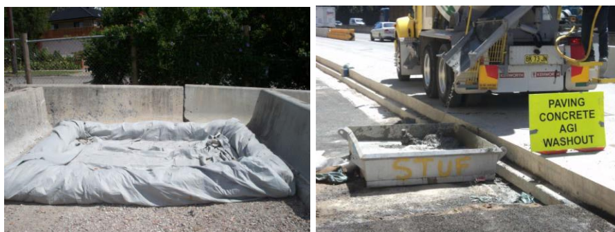
Figures 4 & 5: Concrete wash out
