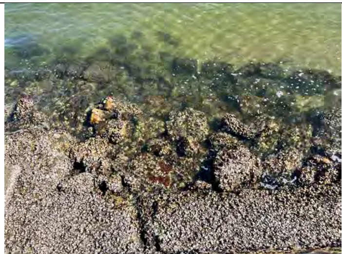
Photo 3 Typical ballast rock / oyster reef.
