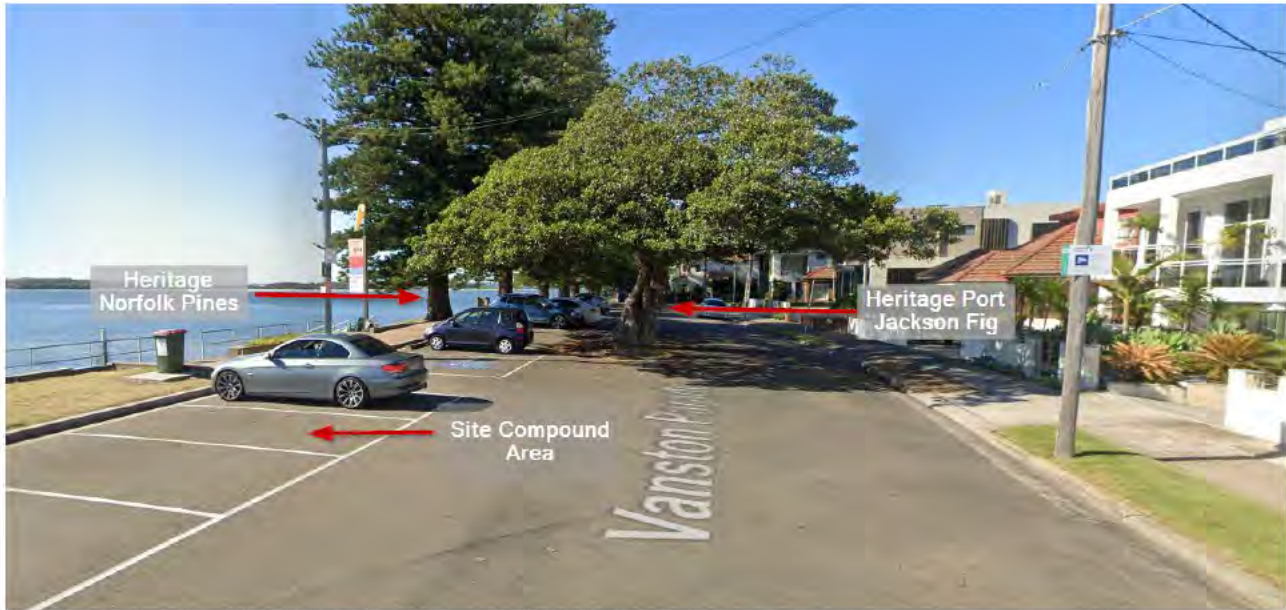
Figure 5-12: View of Vanston Parade (Source: Google Street View, February 2022)
