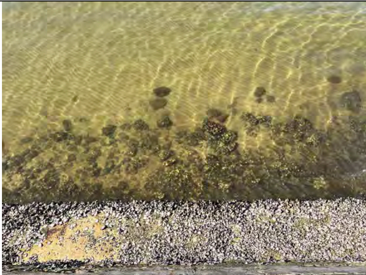
Photo 5 Seawall footing towards the northern end.
