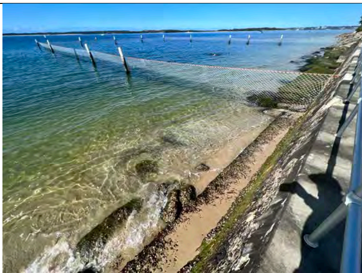
Photo 11 Tidal pool to the south.
