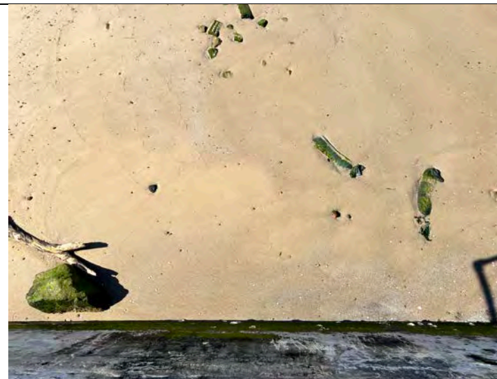
Photo 8 Beach front at base of wall.
