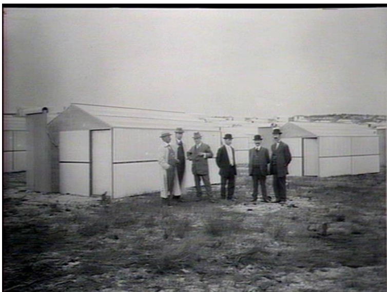
An official inspection of Calico Town. 30
