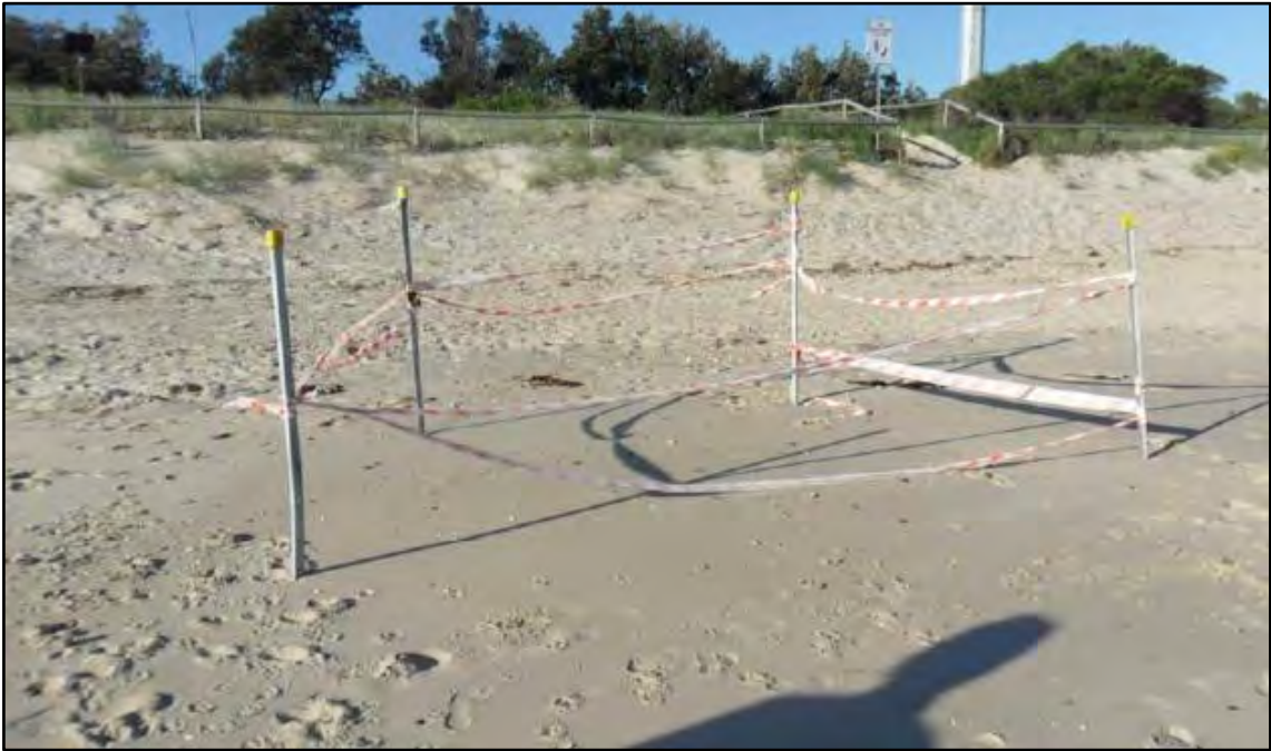
Figure 1-7 Assumed location of blocked Chelmsford Avenue Drain
