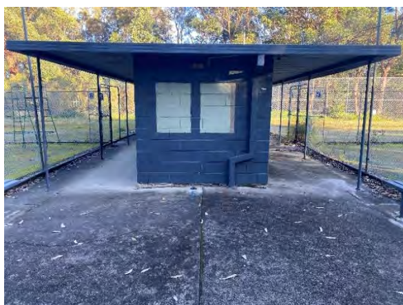
Figure 3-13: View west, showing spectator area and building built onto concrete slab
