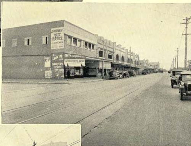
At Right—Gardiners Road, part of shopping centre.
