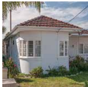
THE PROJECTING CURVED BAYS AND WINDOW DETAILS of 41 Hollywood Street (ABOVE), 71 Culver Street (OPPOSITE) and 79 Hollywood Street (BELOW) illustrate the variety of the Fibro Moderne style. Photographer: Russell Workman 2013.
