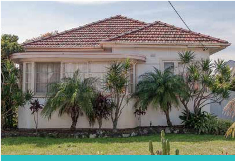
49 CULVER STREET. The curved fibro-cement panels were factory-moulded for ease of installation. Photographer: Russell Workman 2013.
