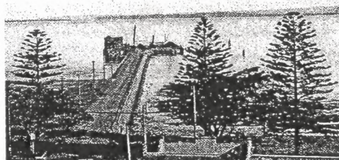
Long Pier Wharf, Botany Bay, c.1938. Built in 1885 for wool cargoes, it was then used for coal loads from 1923 and later demolished during the development of Port Botany. City of Botany Bay Library Service.
