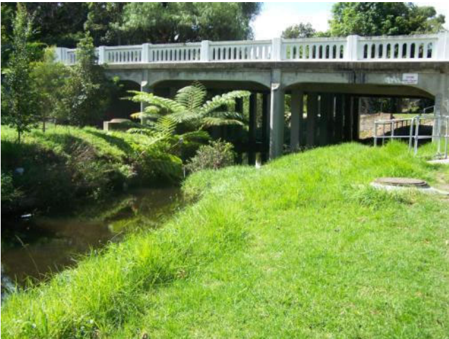
Figure 10 - Bardwell Valley – CFCO Work
