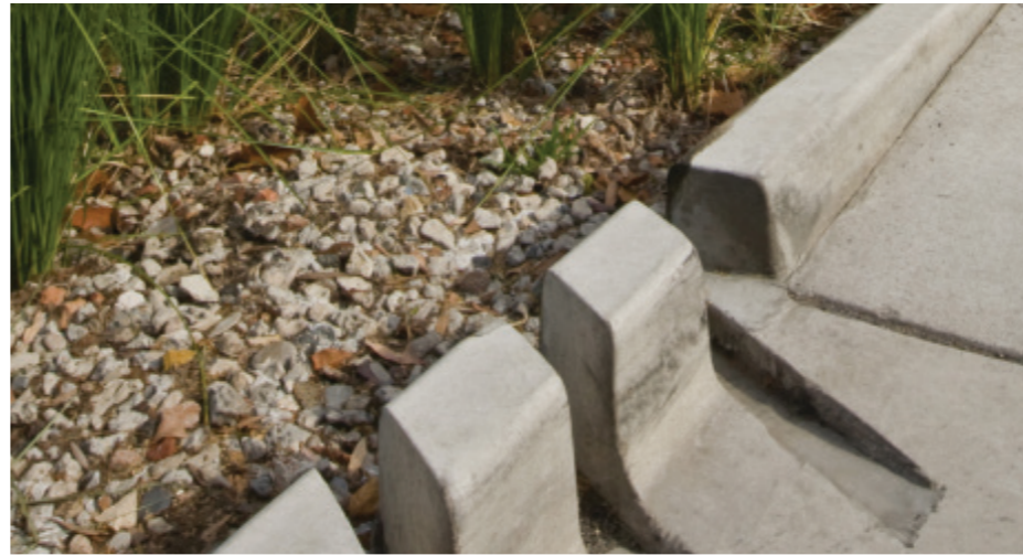
Inlet kerb allows stormwater to be directed to bioswales
