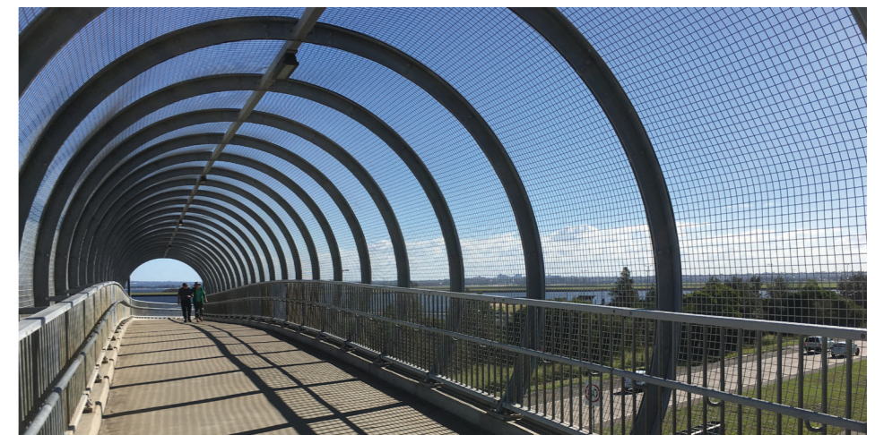
Pedestrian bridge over Foreshore Road
