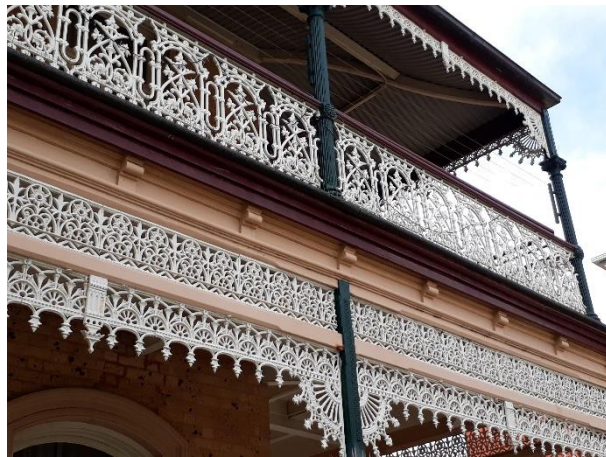
The upstairs balcony features a slatted timber floor and delicate iron lace balustrades.
