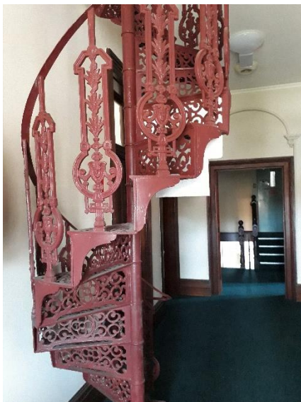
The cast-iron spiral staircase once led to the roof lookout.
