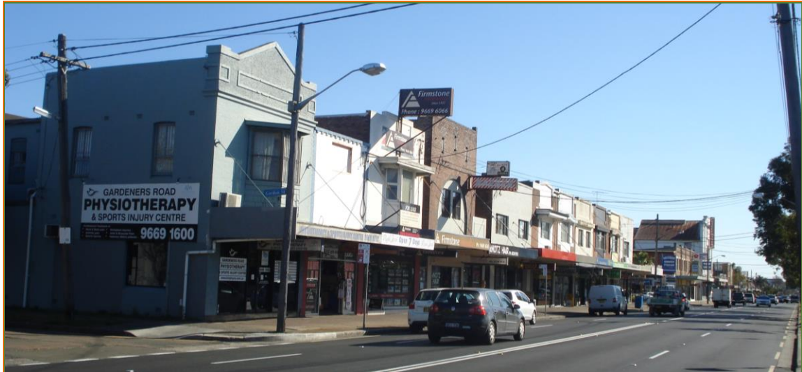
Photo 5 - Rosebery Neighbourhood Centre
