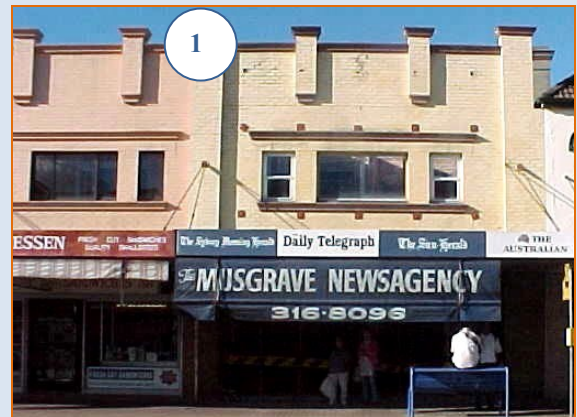
Figure 18 - Decorative Parapet Detailing, which is Found on Two Buildings
