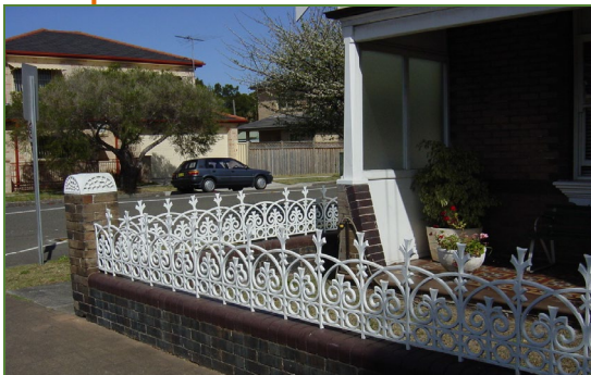
Figure 8 - Original ironwork on brick wall forms an important character of front site.
