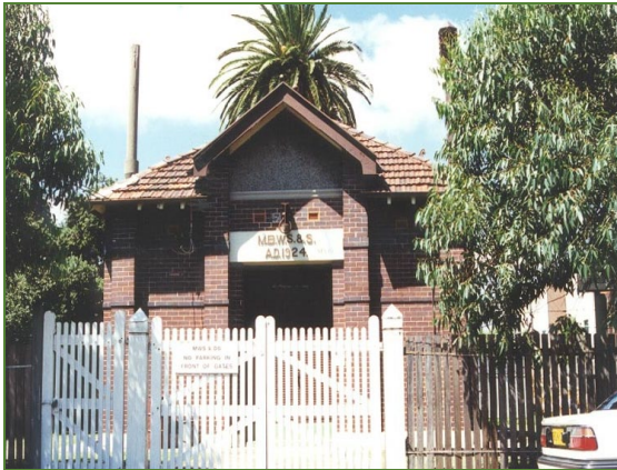
Figure 20 - Pumping Station, Coward Street
