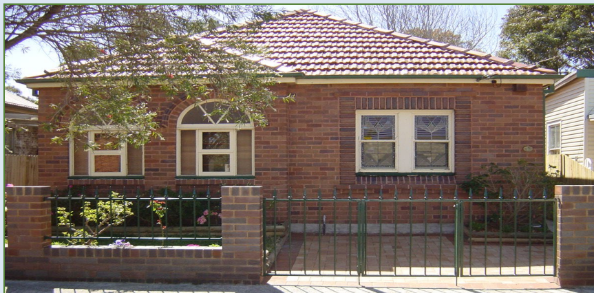
Figure 3 - A Simple Hardstand Area Used to Accommodate a Car
