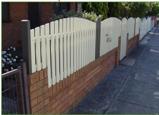
Figure 6 - Original brick fence retained having modern picket fence above
