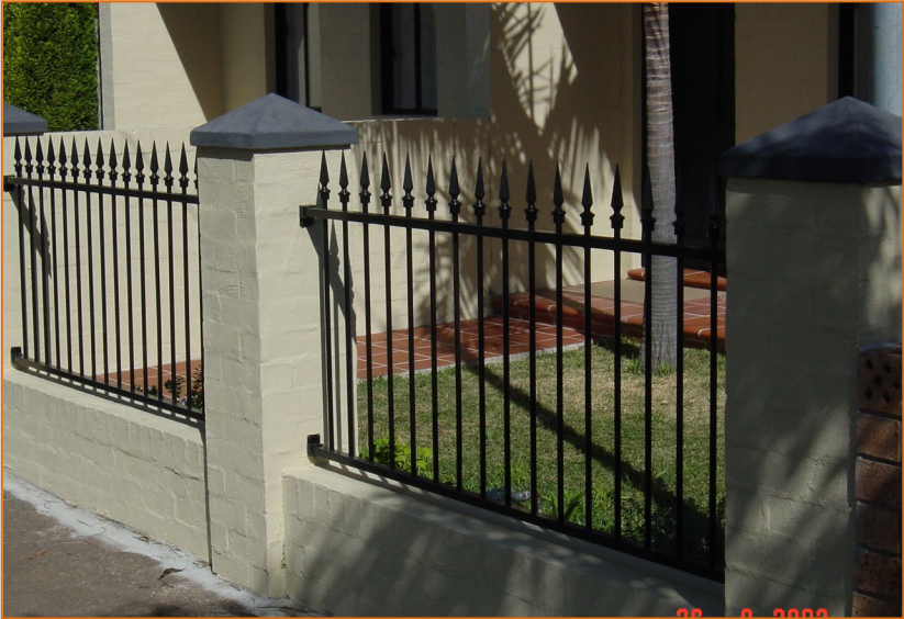
Figure 37 - Example of a Contemporary Fence Suitable for Use Next to Heritage items
