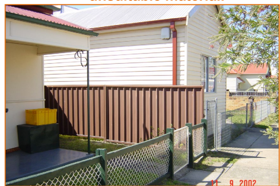
Figure 11 - An example of a fence that is too high in front of the building line and of an unsuitable material.
