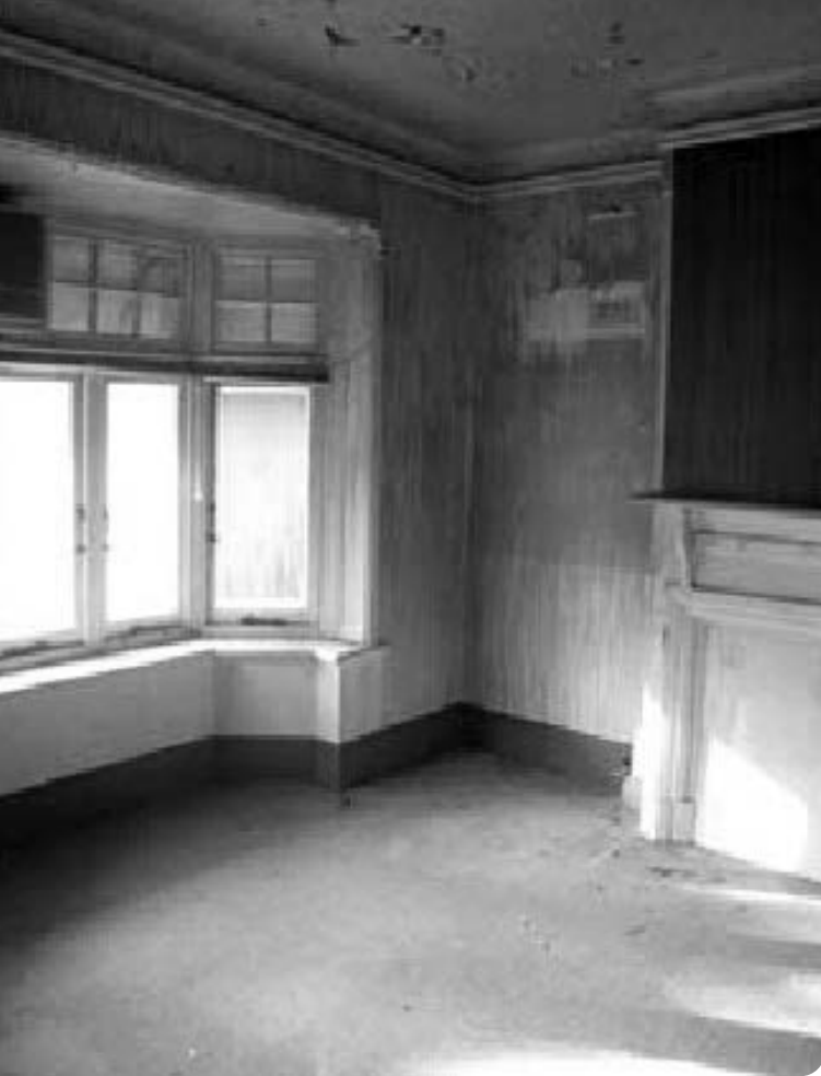
This photograph illustrates the timber bay window, timber fire place surround and timber skirting boards that remain. Source HBO+EMTB (Heritage) 2008
