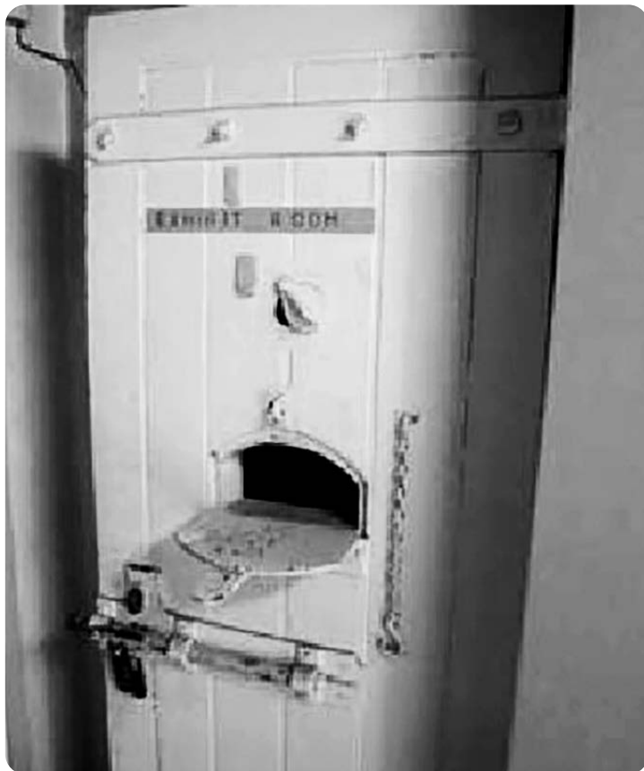
Photo looking at cell #2, main security door with operable meal tray ledge and pivoting peep hole mechanism. Source HBO+EMTB (Heritage) 2008
