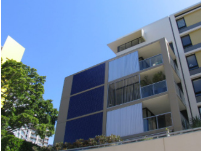
Operable louvres provide climate control
