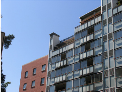
Loggias provide protection from road noise
