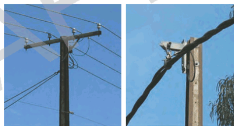
Example: Potential to adapt existing multiple conductors and services lines (left) to insulated aerial bundle cables (ABC)
