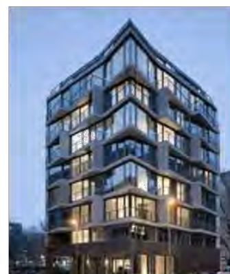
Figure 48: Nine storey apartment building, Berlin Source: www.sustainablecitiescollective.com
