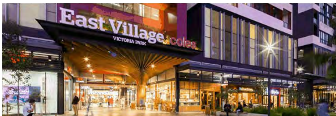
Figure 35: East Village mixed use development Source: payce.com.au
