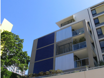
Operable louvres provide climate control
