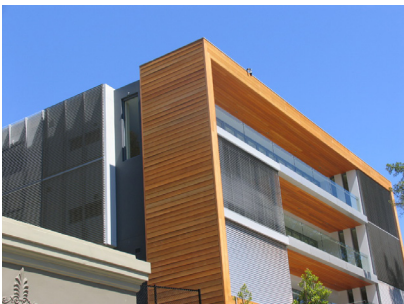
Deep ledges protect glazing from energy loss and gain
