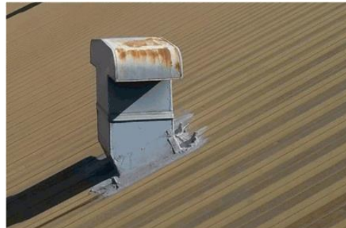
Example of roof penetration showing lack of flashings and previous attempts of repair
