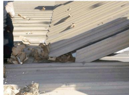
Poor lapping between roofs creating space for leaf debris to accumulate
