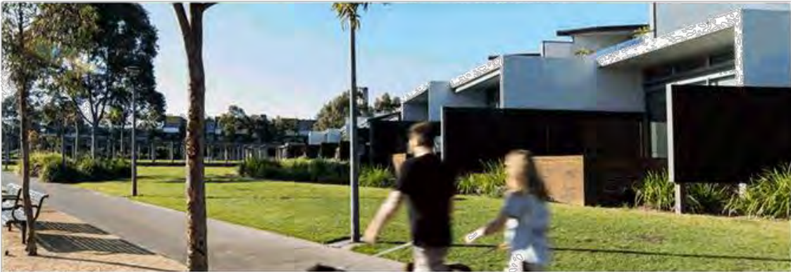
Glebe Harbour Apartments, Glebe
