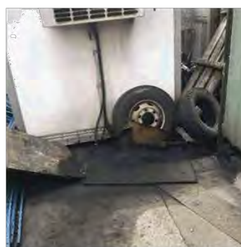
Photo 12. Hydrocarbon stains observed within UST dipping point surroundings.
