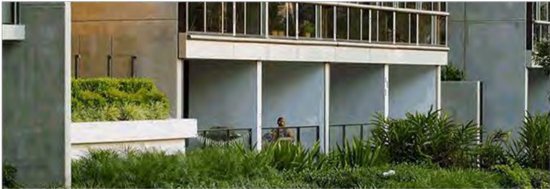
Park Lane, Chippendale (Source: JPW)
