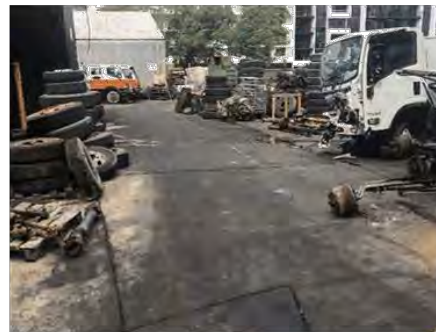
Photo 16. View of concrete slab. Cuts and hydrocarbon stains can be observed.
