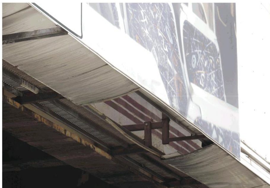
Figure 6: Damage to Sign B
