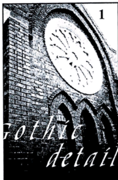
1. Wheel window feature & triple gothic style windows - note cross detail of bricks in the front buttresses. 2. Gothic interior door from porch - etched in memory of Mrs Laurel Goldrich, 1958. 3. Stained glass windows - in memory of Rev. S.S. Horner, 1950. 4. Gothic style entrance door of porch.
