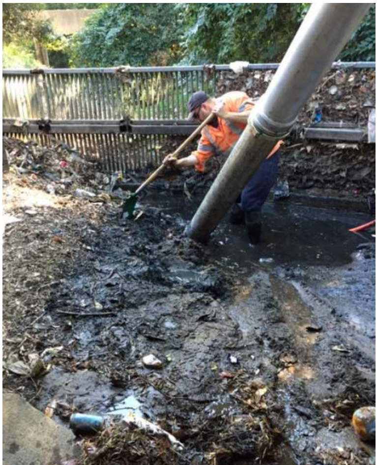
Removing waste from a Gross Pollutant Trap in Bexley
