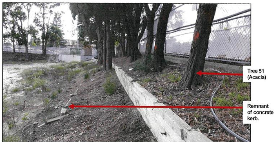
Photo C: Acacia and Casuarina trees proposed to be removed. Remnants of the concrete kerb of the former Carpark are indicated.
