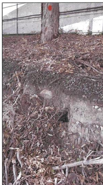
Photo B: Gravel and bitumen surface layer indicating former Carpark level.
