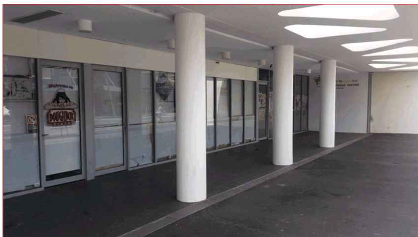
Photo 2.1 Vacant Shop Tenancies in Bay Street
