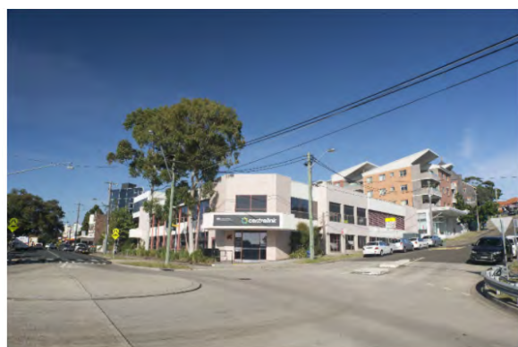
07_ VIEW WEST FROM RAILWAY STREET
