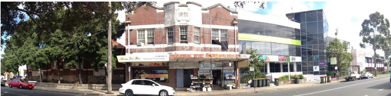
Figure 2 : Photograph of 75-81 Railway Street, Rockdale (Source: G Cirillo)
