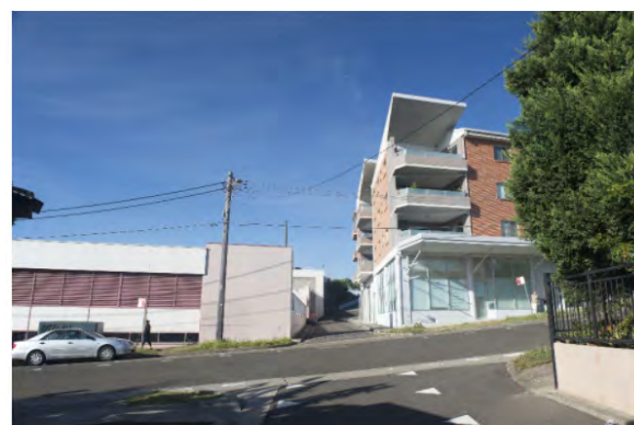
08_ VIEW SOUTH ALONG HESTEN LANE
