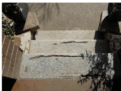
Figure 29 – Detail of the deteriorated terrazzo treads.
