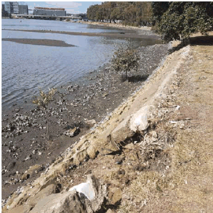
3 - Significant failure at approximately CH 290 in low tide also showing juvenile mangrove establishment.
