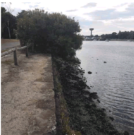
3 - Steep terraced brick wall with mature African Olive tree growing through the wall.
