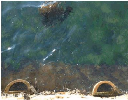
Example of habitat pots able to be retrofitted on seawall providing tidal pool habitats and crevices.
