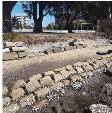
4 - Interface of Reach 3 and Reach 4 where wall is deteriorated, and casuarinas are growing outward towards the river.
