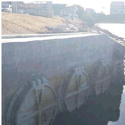
3 - Large stormwater outlet flaps with tidal gates at approximately CH 720
