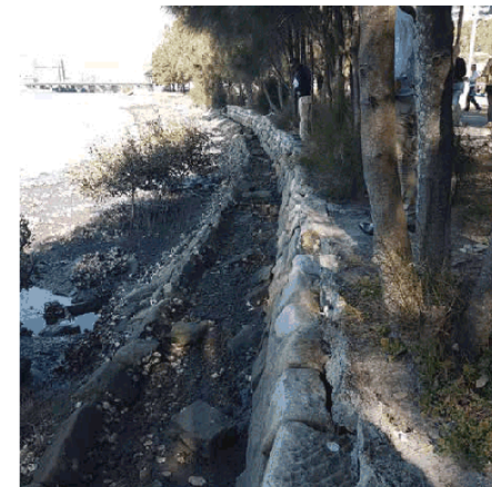
2 - Benched seawall with scattered juvenile mangroves established on the river bed. The stormwater pipe outlet with anti-backflow device (CH381) is visible in the foreground.
