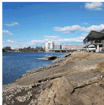
1 - Upstream end of Reach 5 showing old and new boat ramps and undermined timber
