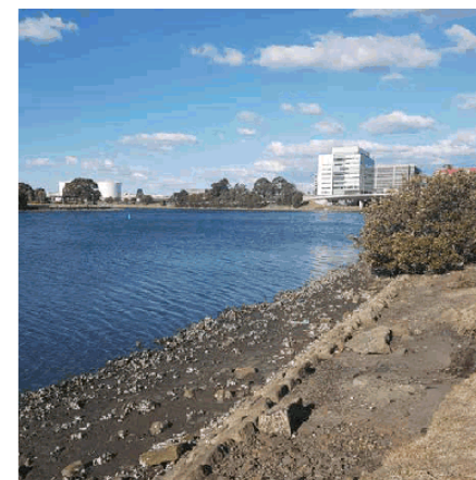
2 - One established mangrove at approximately CH 600 and eroded banks where seawall has failed.
