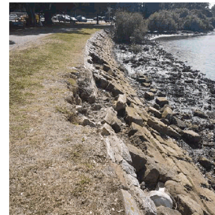
2 - Significant failure at approximately CH 260.
