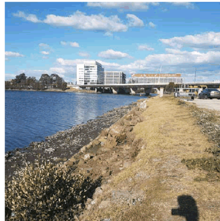
4 - Building rubble and riprap sandstone boulders placed on bank to protect from erosion.
