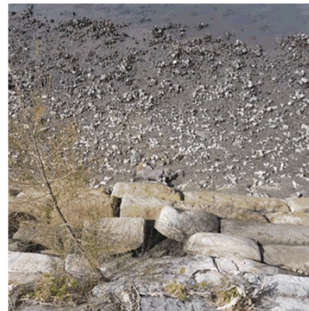
1 - Localised block failure where cauarina shoot has protruded through the wall.
