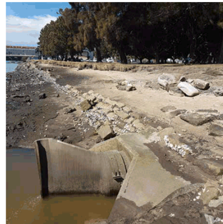
1 - Local stormwater outlet with Tidelflex valve at chainage 425.
