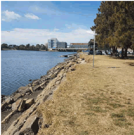
3 - Small section of intact seawall between CH 500-520.
