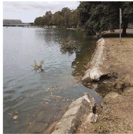
4 - Significant failure at approximately CH 290 in high tide
