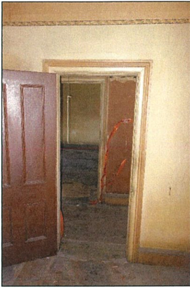
Figure 47. View to Lounge room door opening (D2). Note painted timber 4-pannelled door.
