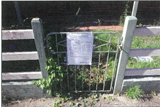
Figure 32. Metal gate in front fence. Element of little significance.
