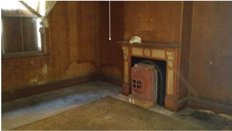
Figure 22 - Fireplace and projecting chimney breast in rear western room (Dining Room).
