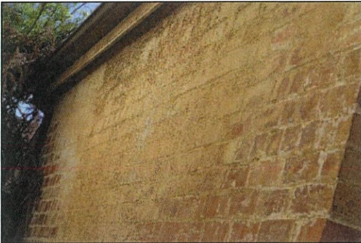
Figure 22. Close-up view of western elevation. Note evidence of previous paint coat.
