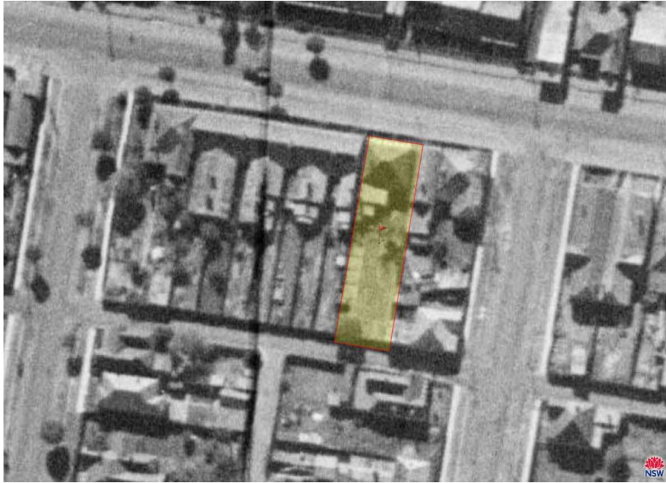
Figure 9 – Detail from 1943 aerial showing subject site shaded yellow. The extent of the original kitchen and outhouse are clearly visible as are the extent and form of the adjoining cottages in King Street. (Source: NSW Land & Property Information, SIX Maps)
