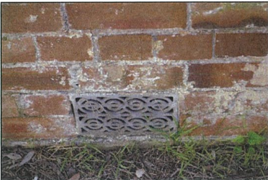
Figure 24. Close-up view of metal verticillation grille to sub-floor, southern elevation.
