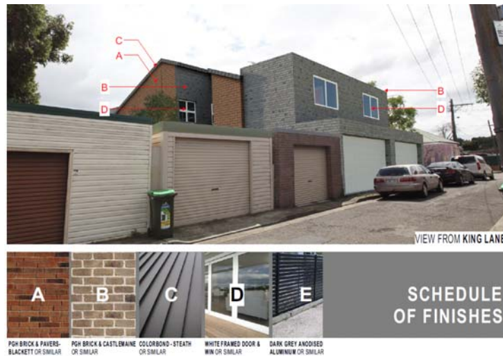
Figure 10: Schedule of Materials and Finishes
