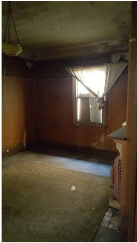
Figure 21 - Rear room western side (Dining Room)
