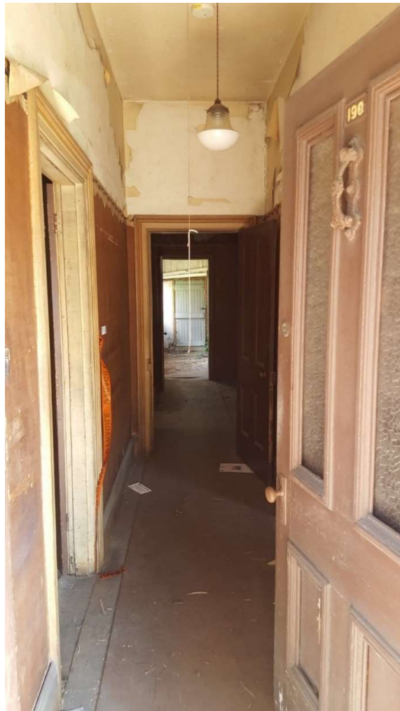
Figure 15 - Front door and entry hall looking through to back door.
