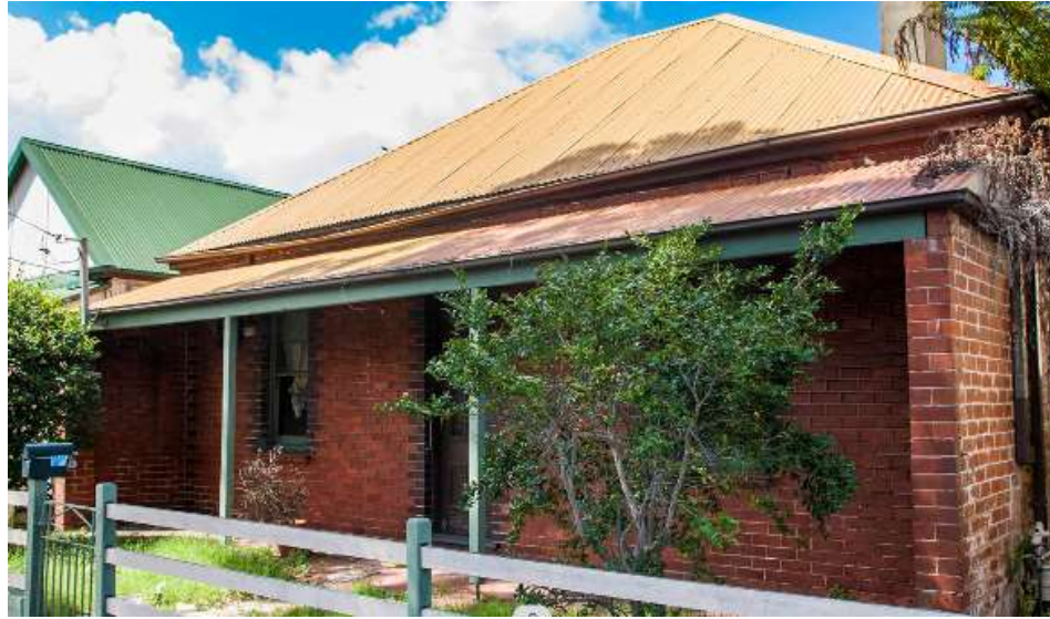
Figure 11 - View of the front verandah showing the face brick fin walls, contrasting brick trims and modern replacement corrugated metal roofing. The verandah posts are modern replacements. The original may have had decorative brackets but these are no longer in evidence. Face brickwork is restricted to the front facade
