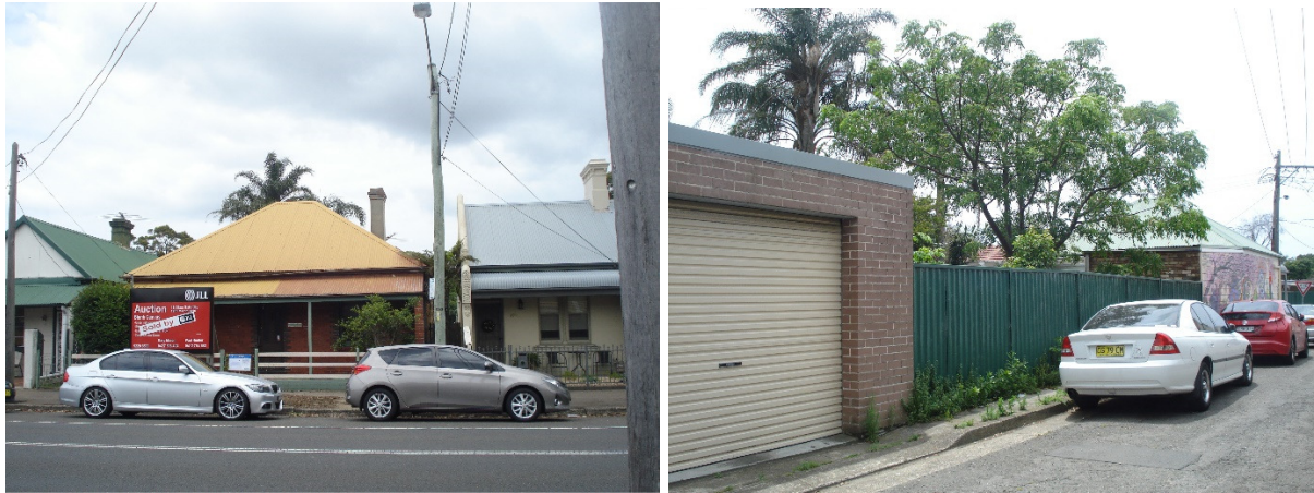
Figure 8: Front and rear view of the subject site
