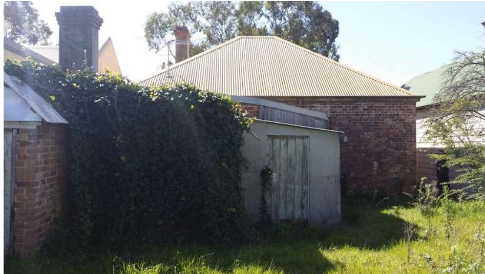
Figure 13 - Rear view of 190 King Street, Mascot showing the rear service areas set under skillion roofs which are proposed to be demolished. The large chimney is the former kitchen fireplace. The rear and side walls appear to be solid 9 inch brickwork with no cavity.
