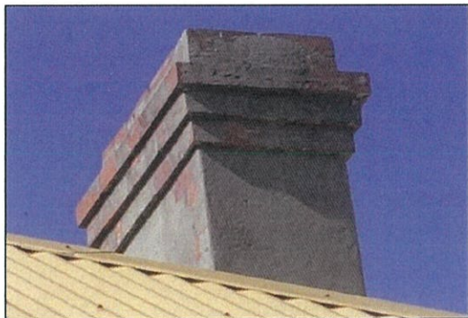
Figure 3. Close-up of chimney. Note evidence of worn render.
