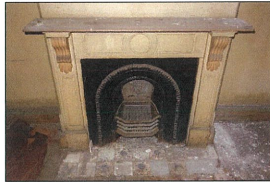
Figure 54. Close-up of fireplace and mantle-piece with original cast-grate and chimney breast, Lounge room.
