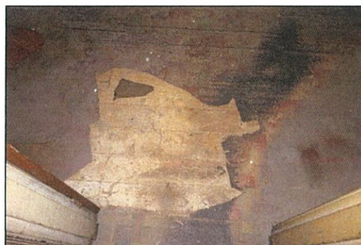
Figure 45. Exposed timber floorboards, Lounge.
