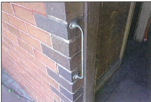
Figure 8. Close-up of later addition metal handrail.
