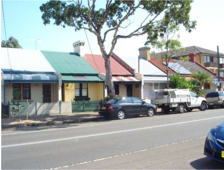
Figure 4 - Group of Victorian era attached cottages King Street Mascot from State Heritage Inventory.
