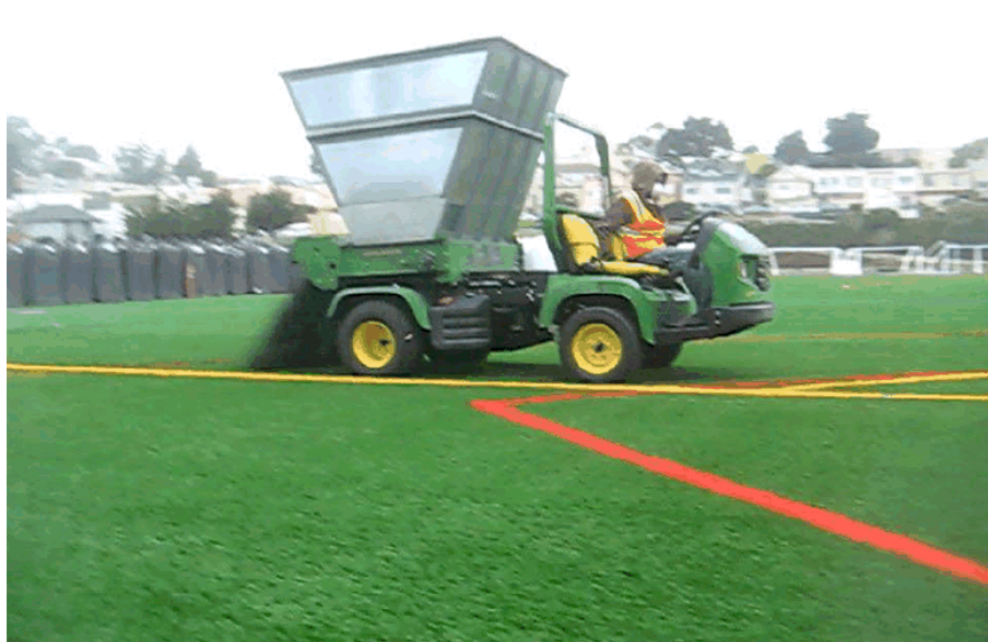
Figure 3.2 Semi-mechanised application of infill
