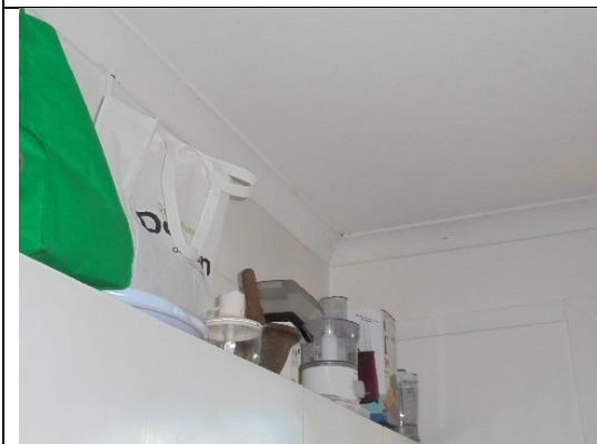
Figure 35 – Ceilings throughout the building were replaced c2000 with painted plasterboard and coved cornices.
