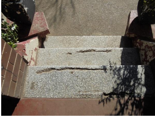
Figure 29 – Detail of the deteriorated terrazzo treads.
