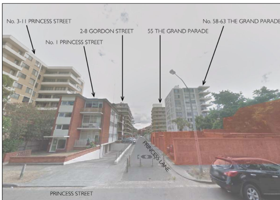
Figure 7 – Photograph showing locations of surrounding properties (Source: Urban Design Report)
