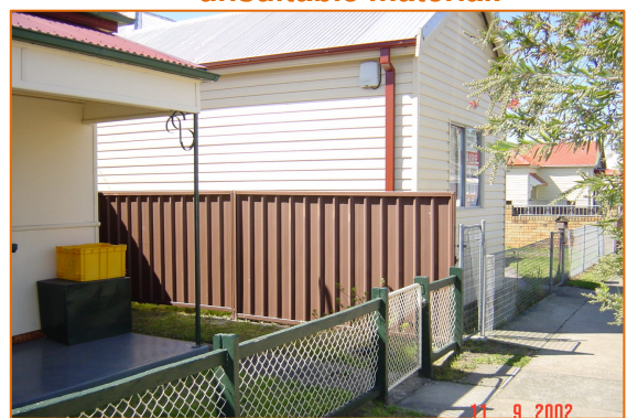
Figure 11 - An example of a fence that is too high in front of the building line and of an unsuitable material.
