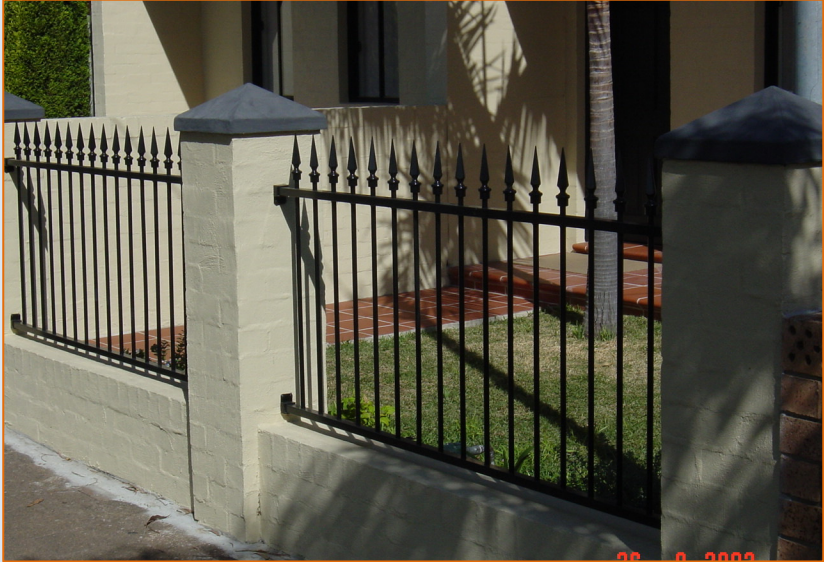
Figure 37 - Example of a Contemporary Fence Suitable for Use Next to Heritage items
