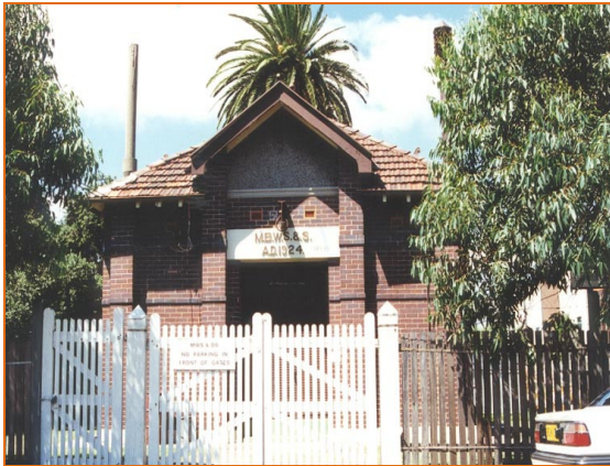
Figure 20 - Pumping Station, Coward Street
