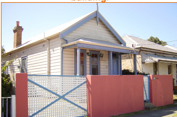
Figure 10 - This fence is too tall the building behind and its solid conceals too much of the building.
