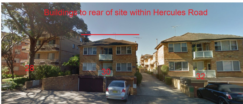
Figure 5 - Hercules Road properties to the rear of the site
