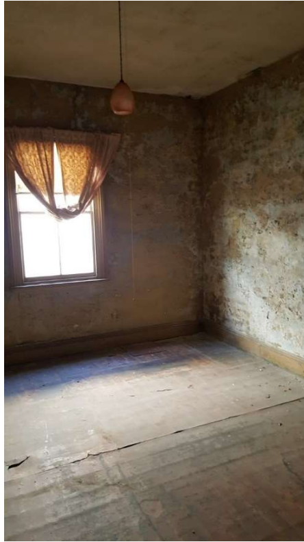
Figure 20 - Front room on eastern side (Bedroom) showing severely deteriorated plaster wall condition.
