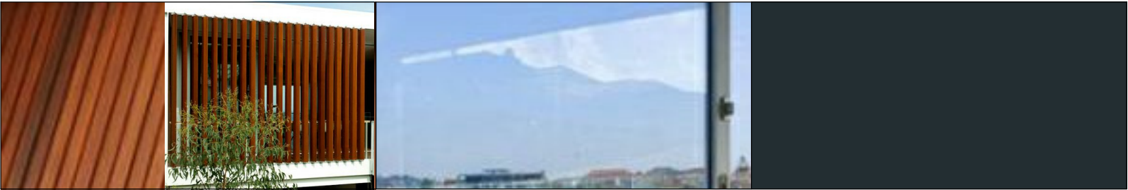
04. DECOWOOD PRIVACY SCREENS WESTERN RED CEDAR VERTICAL FIXED LOUVRE PRIVACY SCREENS TO BE POSITIONED AND ANGLED TO OBSTRUCT POTENTIAL VIEWS ONTO NEIGHBOURS 05. GLASS GLASS WINDOWS & DOORS CLEAR GLASS 06. WINDOW FRAMES ALUMINIUM WINDOWS AND DOORS MONUMENT
