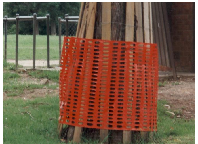
Photo 18: This serves little purpose at all! It does not protect the roots or the trunk of the tree.
