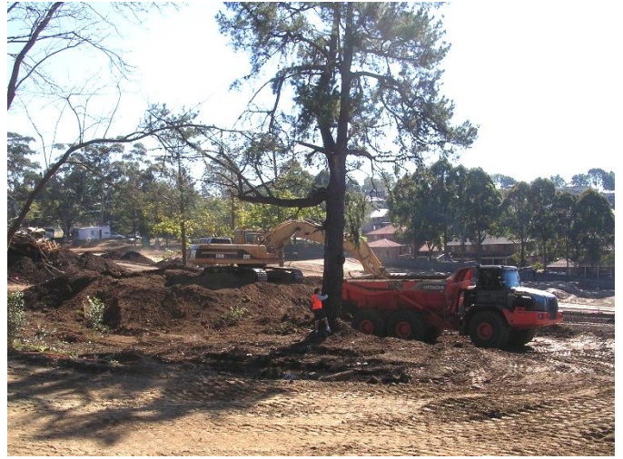
Photo 8: A single movement of a truck can cause significant damage to the absorbing roots.
