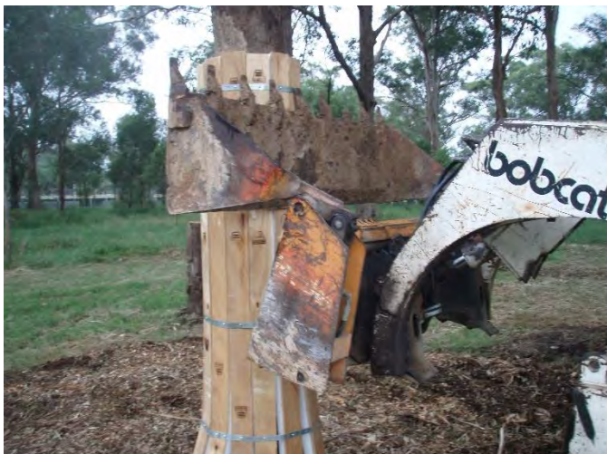
Photo 17: Able to withstand and absorb moderate construction impact - not that this should happen!
