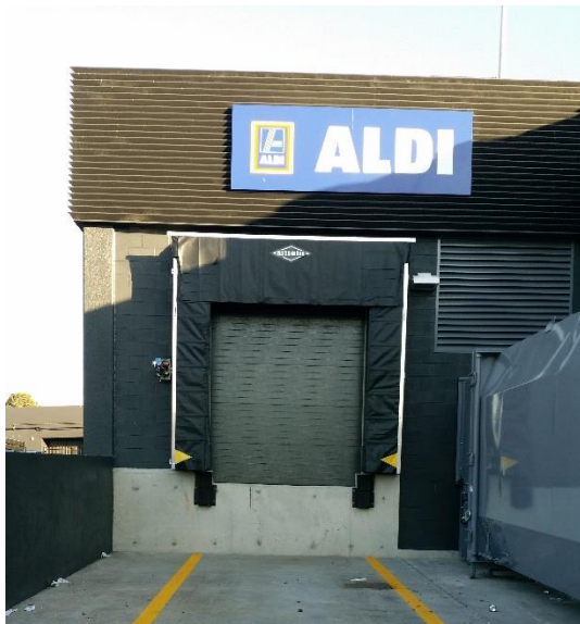
Photo 1: Loading Dock Curtain to the Southern Loading Dock
