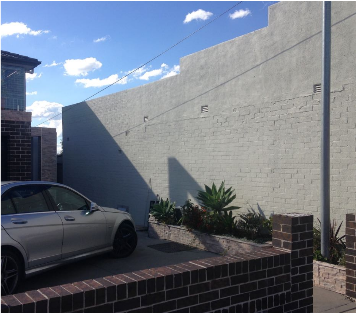
Figure 3: Part of the front setback area of 40 Stoney Creek Road, with the side wall of the existing building on the subject site visible
