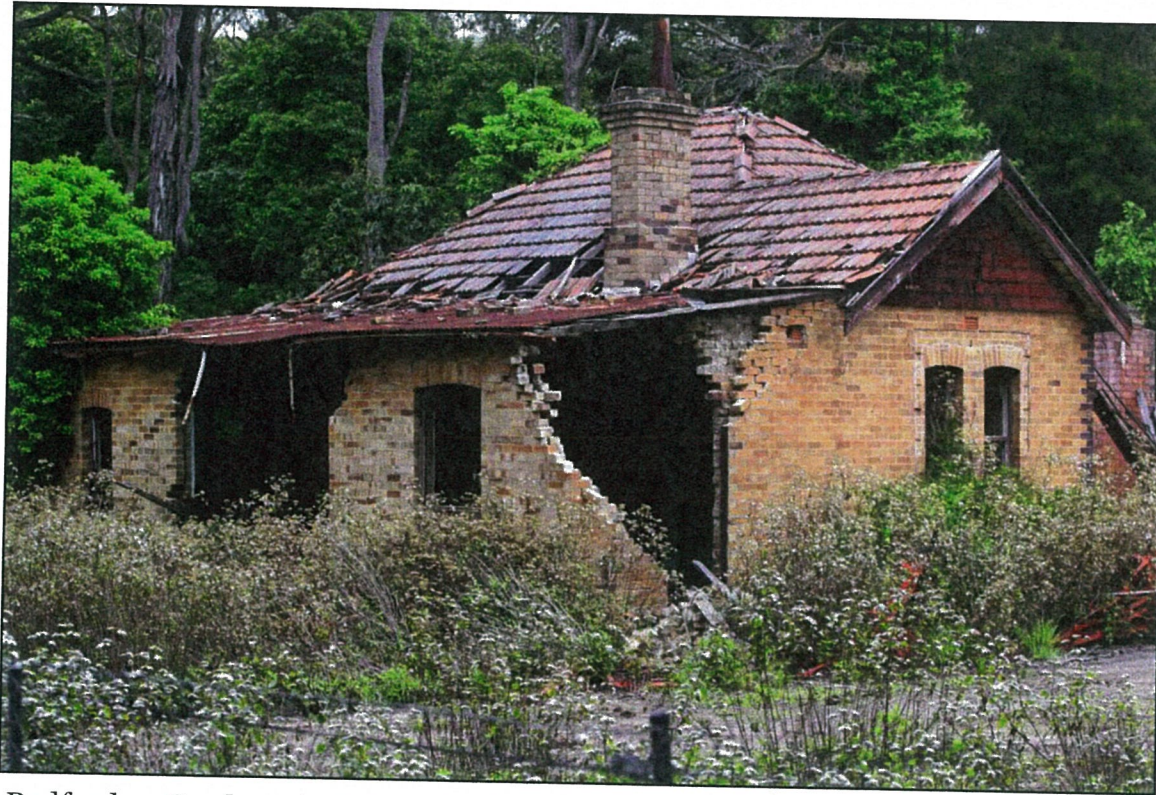
Bedford or Gardener's Cottage built by James Toyer c 1915 and demolished 2013. This served as the centre of the Toyer transport operations in the Royal national Park and was situated near the Prince's Highway at Loftus.
