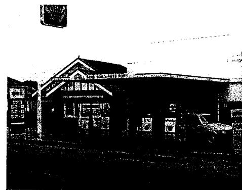
James Toyer's home and service station on the corner of Rocky Point Rd and Evans St., Sans Souci.
