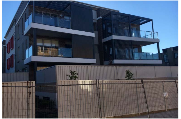
Site Inspection Photo 6 – Viewing adjoining development at 690 Princes Hwy from Cross Lane (rear of subject site).
