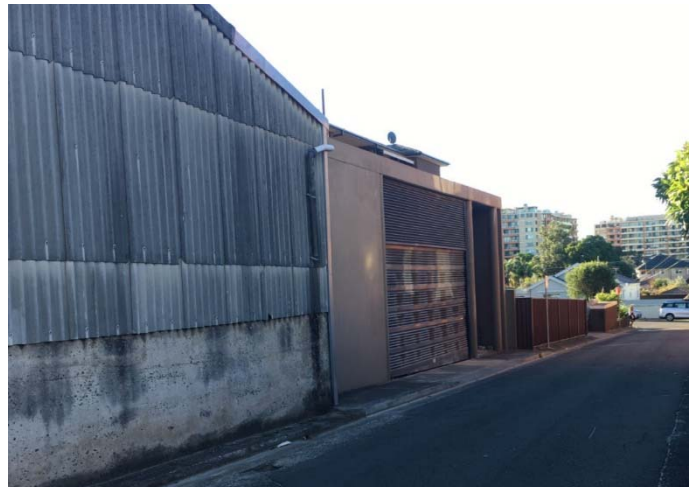
Site Inspection Photo 8 – Viewing part of the rear of subject site (building with corrugated sheeting) and adjoining development at 684 Princes Hwy from Cross Lane.
