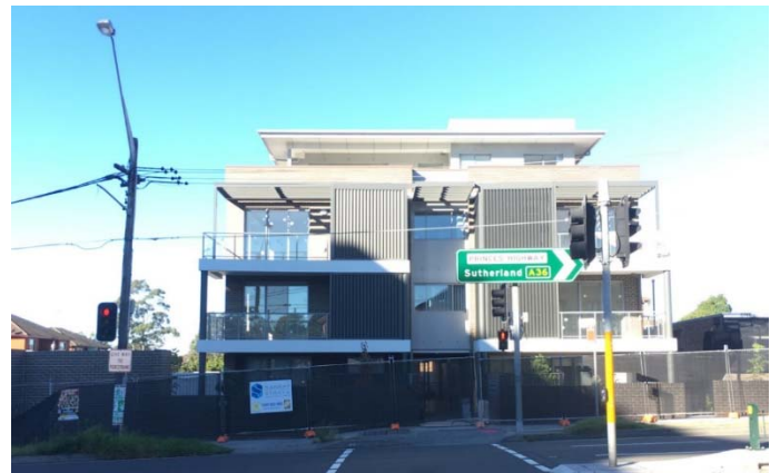
Site Inspection Photo 2 – Viewing adjoining development at 690 Princess Hwy (under construction).
