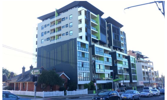
Site Inspection Photo 4 – Viewing recently constructed development at 29-31 Princess Hwy, located north-west of the subject site within the Georges River Council local government area.
