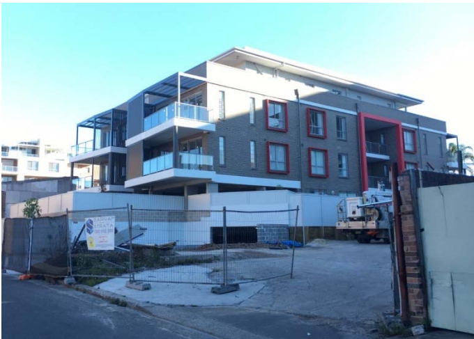
Site Inspection Photo 7 – Viewing rear of subject site and adjoining development under construction at 690 Princes Hwy from Cross Lane (rear of subject site).
