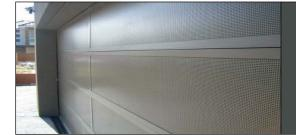
10. GARAGE DOOR PERFORATED ALUMINIUM POWDER COATED ASTRO
