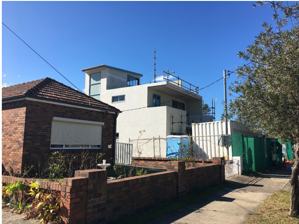
Example of a poorly located and designed awning in comparison to our proposal, facing the side boundary neighbour at nearby 9 Robinson Street
