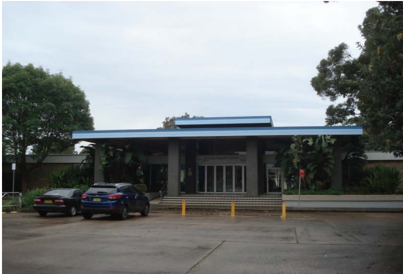
Figure 6. Botany Aquatic Centre 50m to the east of the existing amenities building
