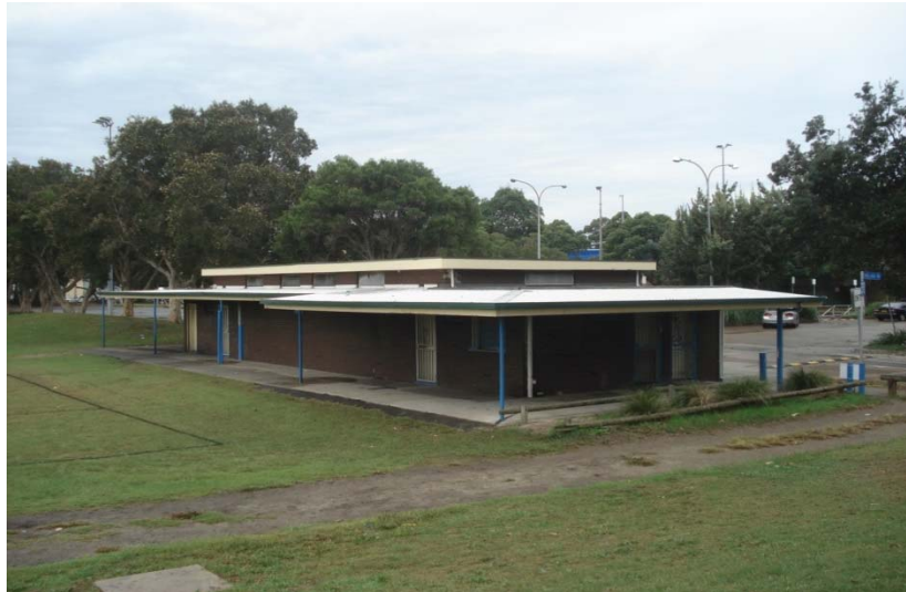
Figure 3. Existing amenities building as viewed from the south-west
