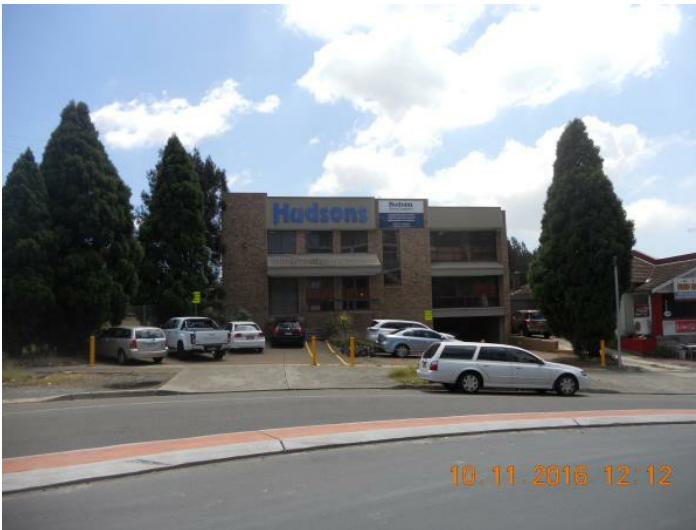
Figure 6 - No. 1 Arncliffe Street (located immediately to the west of the site)
