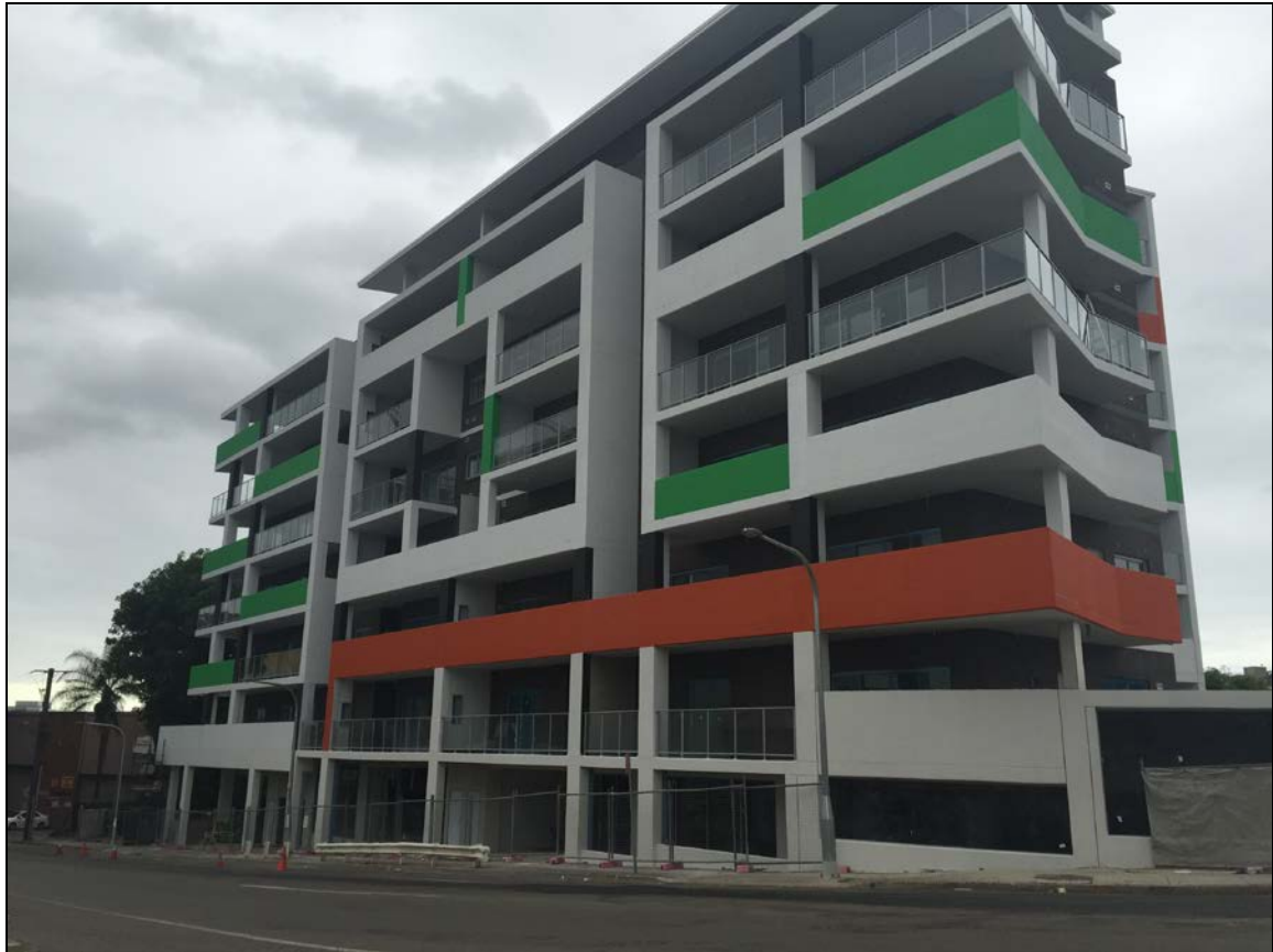
Figure 4: view of the development under construction to the south of the site, looking south east from Arncliffe Street
