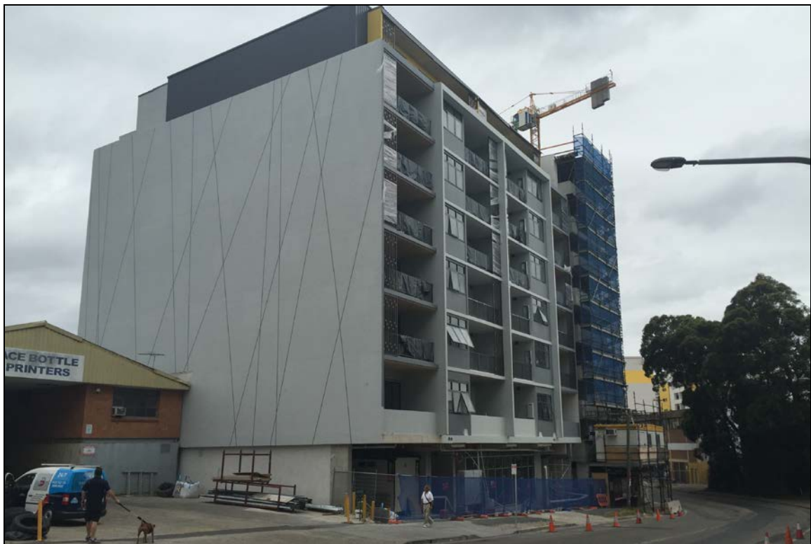
Figure 6: View of Nos 9-11 (in the foreground) and 13-21(behind scaffolding) Arncliffe Street, looking north east from Arncliffe Street
