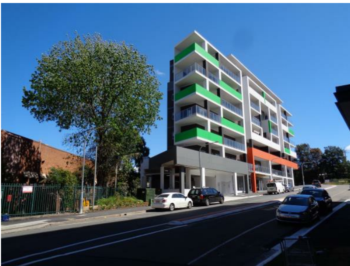
Figure 9 - No. 30-32 Arncliffe Street, located opposite the subject site.
