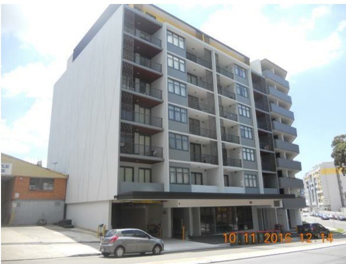
Figure 8 - No. 9-11 Arncliffe Street
