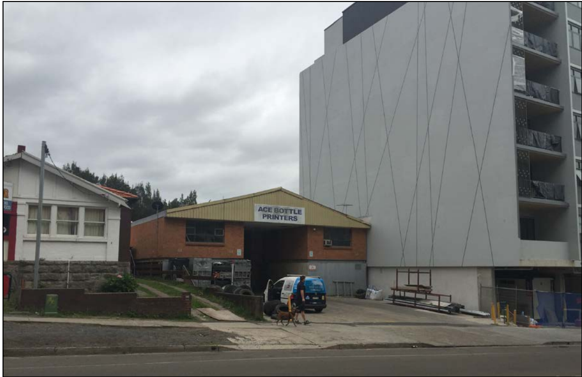
Figure 5: View of No. 7 Arncliffe Street, looking north from Arncliffe Street
