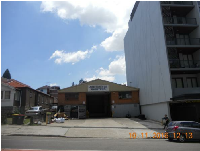
Figure 7 - No. 7 Arncliffe Street (& 9-11 Arncliffe Street, Wolli Creek), located immediately to the east of the subject site.
