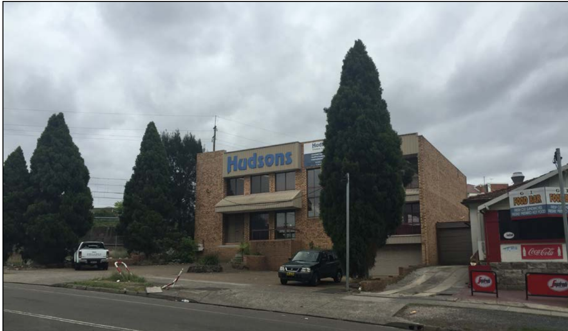
Figure 7: View of No. 1 Arncliffe Street, looking north west from opposite the front of the site
