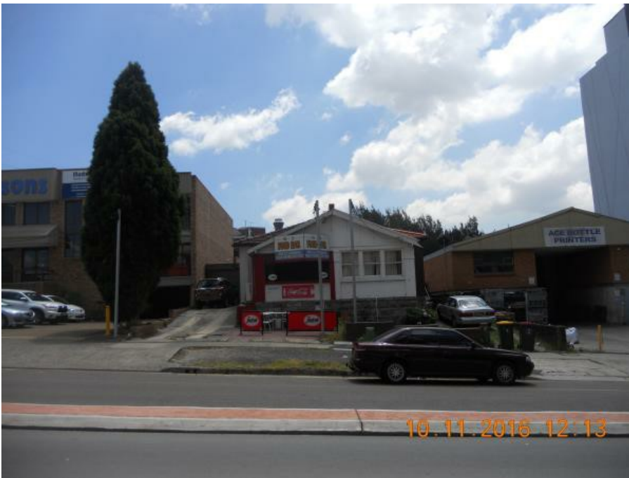
Figure 3 - Subject Site (3-5 Arncliffe Street), and part of adjoining sites No. 1 & No. 7 Arncliffe Street
