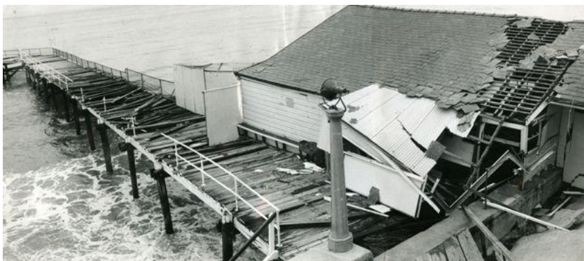
May 1968 Storm damage to Brighton Baths. Photo: Bayside Council Library
