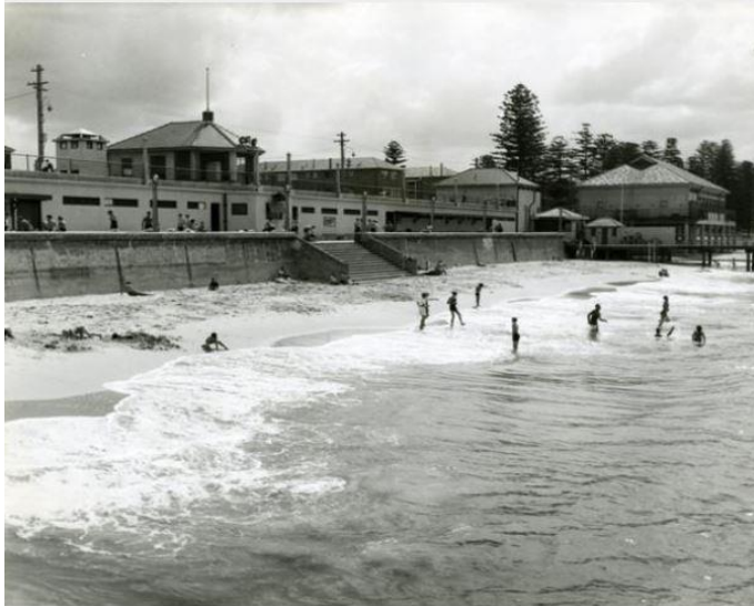
Brighton Baths pavilion and dressing sheds 1950s. Photo: Bayside Council Library.
