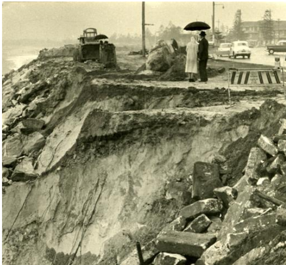
1966 Storm Damage to Cook Park, alongside The Grand Parade, nearly destroys a section of road.
