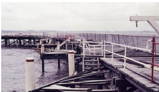
Storm damage to Brighton Baths, 1965. Photo: Bayside Council Library
