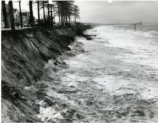
Storm Damage to Cook Park 1966. Photo: Bayside Council Library
