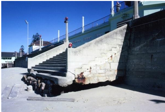
Storm damage to Brighton Baths stairs, 1962. Photo: Bayside Council Library
