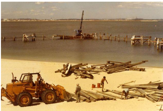
The demolition of Brighton Baths, 1978. Photo: Bayside Council Library
