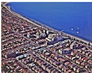
A 1980s aerial photo of Brighton Le Sands near the intersection of Bay Street and The Grand Parade, showing Lady Robinsons Beach and the construction of the Novotel Hotel Photo: Bayside Council Library
